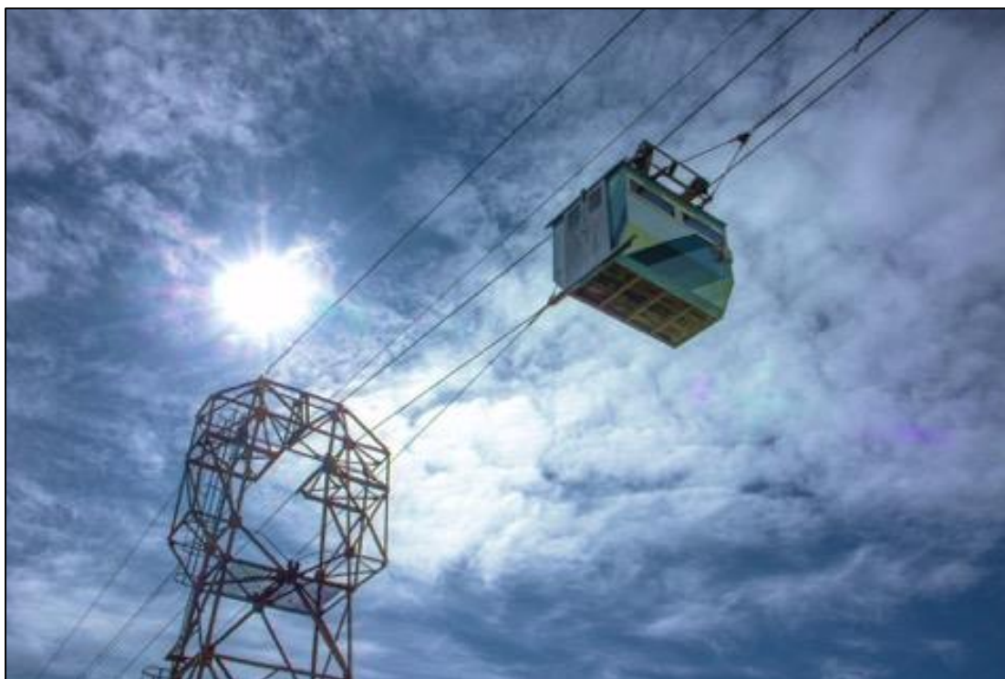
Plate 2.2 Portion of existing cableway infrastructure, including the cable car and the pylon
