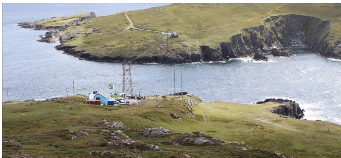
Plate 2.1 Existing Dursey Island Cableway and site of proposed development
